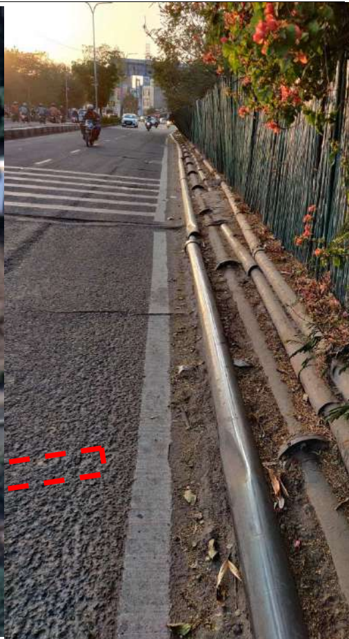
Figure 14: Exposed Underground Utilities
