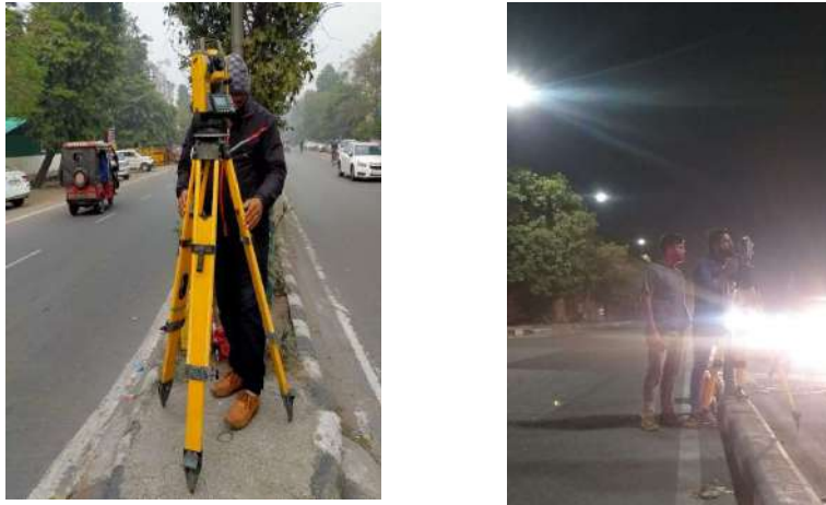
Figure 25: Total Station Survey image
